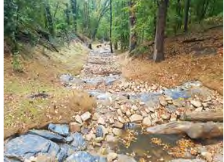
Regenerative Stream Conveyance (RSC) - "Step Pools" to slow runoff, filter water by allowing to percolate into the ground, and reduce sediment flows
