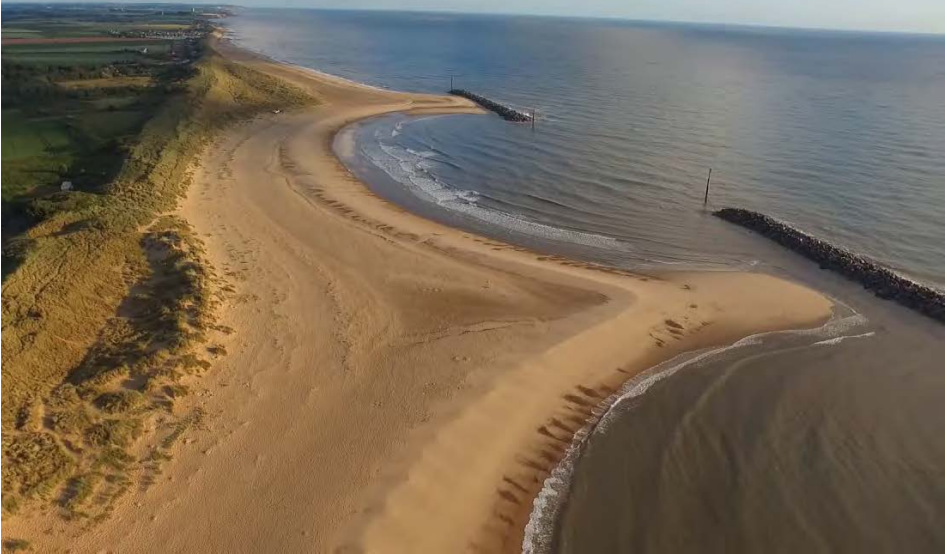
Living Shorelines utilizing Offshore Breakwaters - Used for high-energy coastal systems to control and dissipate wave energy in order to increase sediment accretion to on beaches
